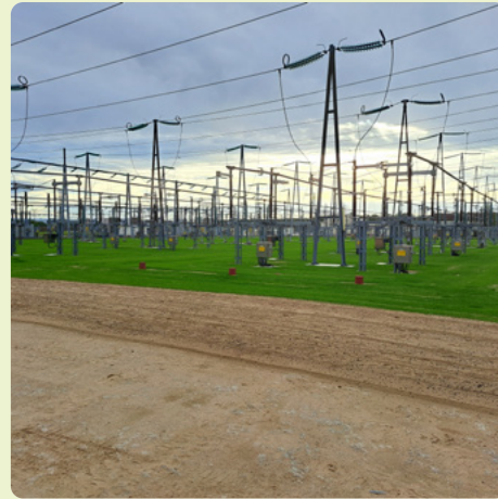
↑ Hydro-mulching near electric sub-stations, France
