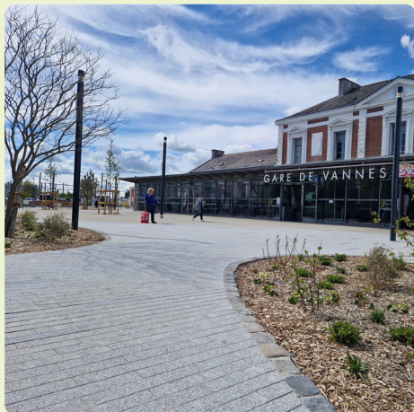
↑ Béton durable, Vannes, France
